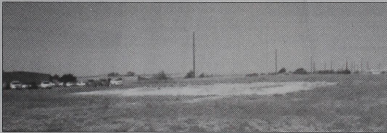
UNDER CONSTRUCTION: The Allison Church of Christ is in the process of having a new church constructed between Ware Chevrolet and Baymont Inn and Suites.
