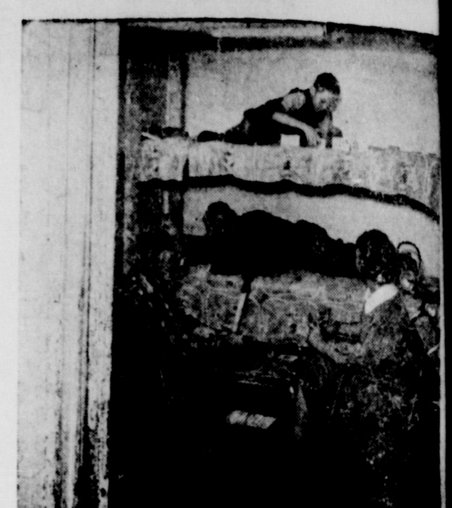
A CLOSE CALL with a tornado in 1953 led the Donald L. family of Toledo, Iowa, to build their own small shelter in their basement. They estimate that, by doing their own work, they will have only about $69 in the shelter when finished. He, son, his wife Jean, and sons Rick, 12, (lower bunk) and 12, "try the shelter out for size." In addition to serving as a tornado shelter, it would be valuable as protection against active fallout if the nation were attacked.
