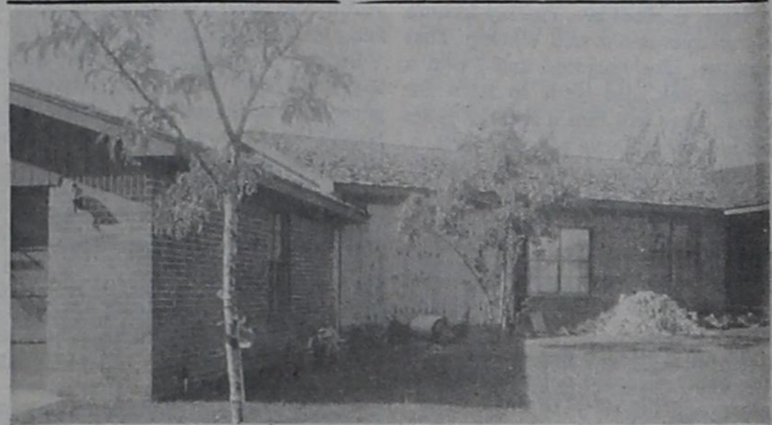
Boarded Up After Accident
