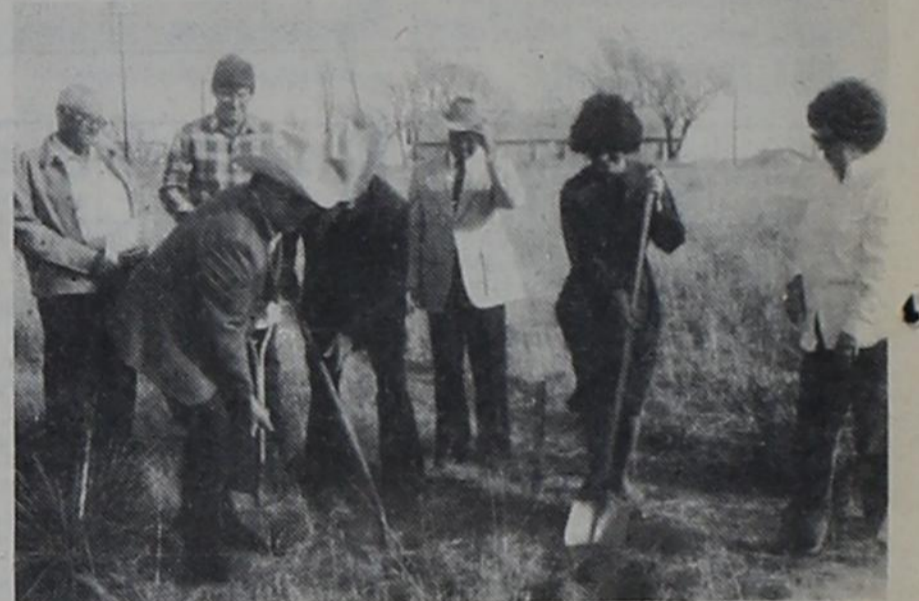
GROUND BREAKING: Richard Kiker, Leonard Powledge and Daronda Begert turn a shovel of dirt at the Groundbreaking Sunday afternoon, November 30, for the Allison Methodist Church. Looking on are George Parker, Alton Lohburger, Bob Zybach and Suzanne Lohburger.
