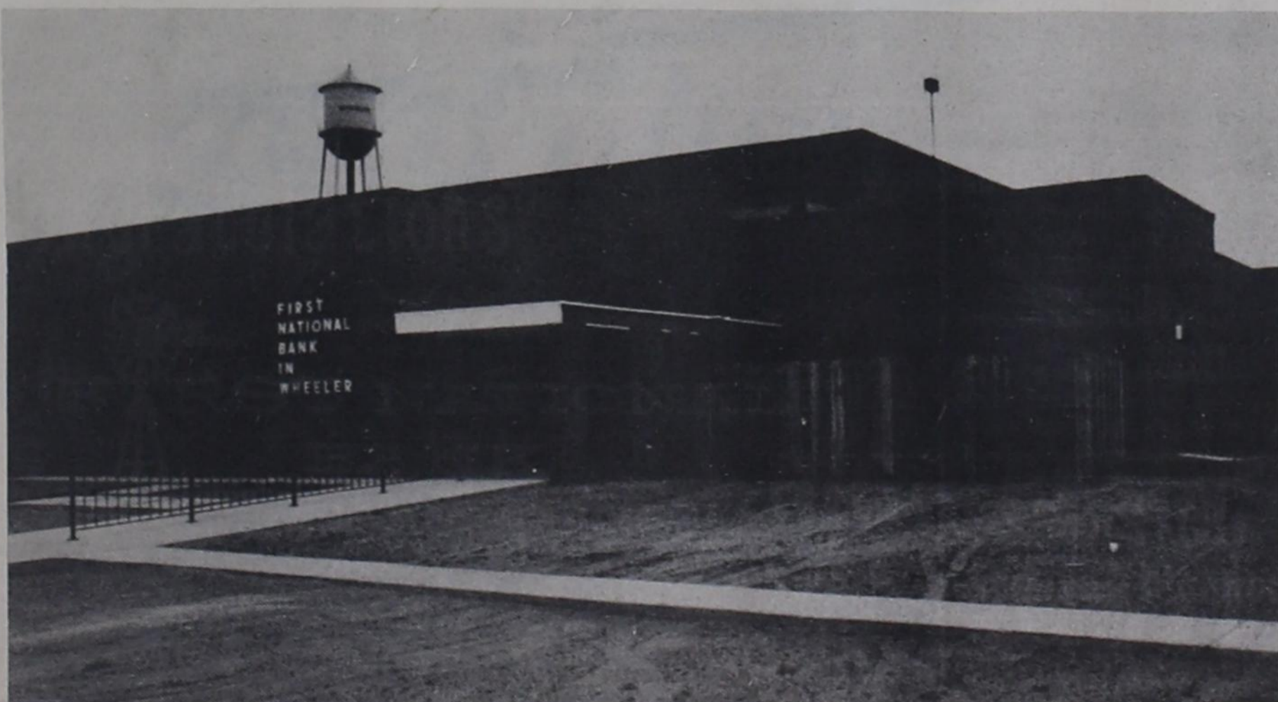
... Back Entrance & Community Room
