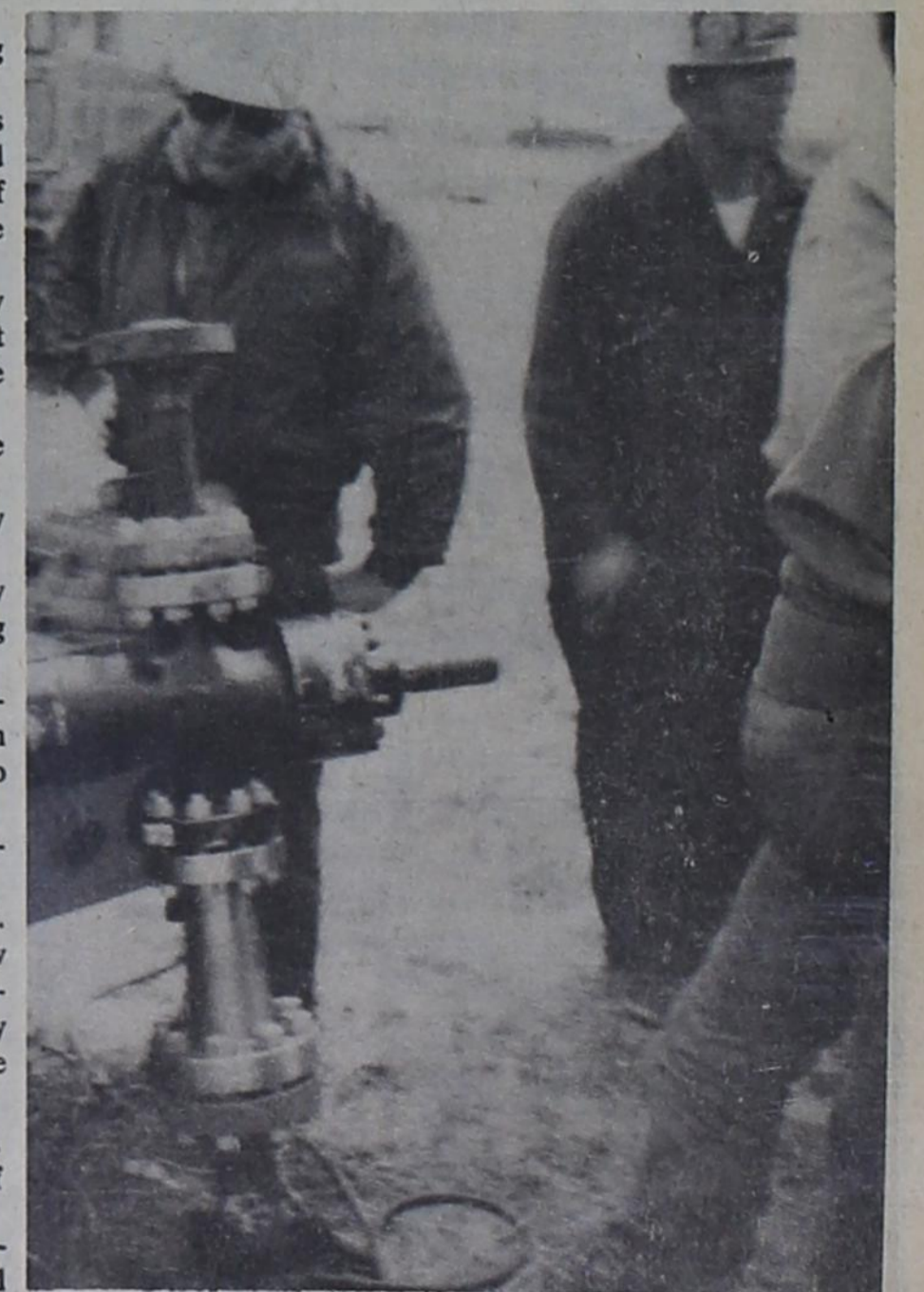
IT DID THE JOB: Red Adair arrived on the scene Wednesday north of Wheeler and assessed the situation. He determined the type valve necessary to cut off the flow of gas and sent to Pampa to have the valve built. The valve shown was put in place and the well was capped Friday afternoon.
