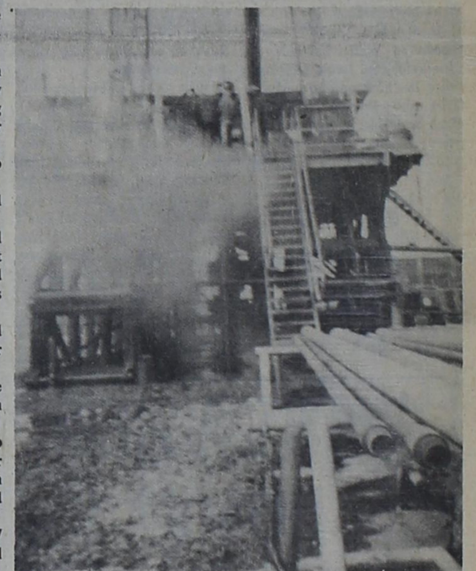
ESCAPING GAS: The Atherton well north of Wheeler is shown here as it looked when Red Adair arrived to begin work. The gas appears as a fog to the left of the picture.
