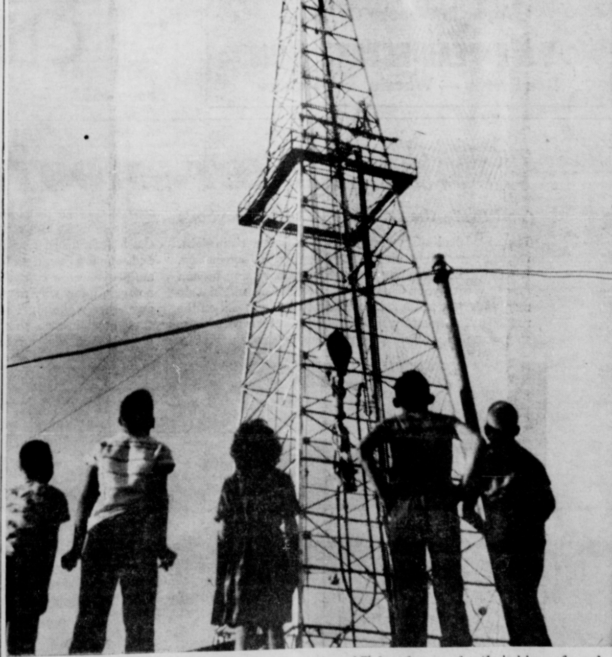
ANOTHER BIG ONE: Parker Drilling Company of Tulsa, famous for their big, safe and well kept rigs, has earned another feather for their cap. This rig located a couple miles West of Reydon, Okla., just over the Texas line, is one of the biggest in this area. The tower is 136 feet; sub-structure 23 feet. And at last report the crew was drilling at 14,807 feet, and was drilling approximately 100 feet per day. Three five-man crews keep the rig in operation 24 hours a day. The well is being drilled by Parker for Gulf Oil. The kiddoes trying to see the top of the rig are: (left to right) Darrell Lang, Don Lang, Becky Vanpool, Darrell Butler and David Lang.
