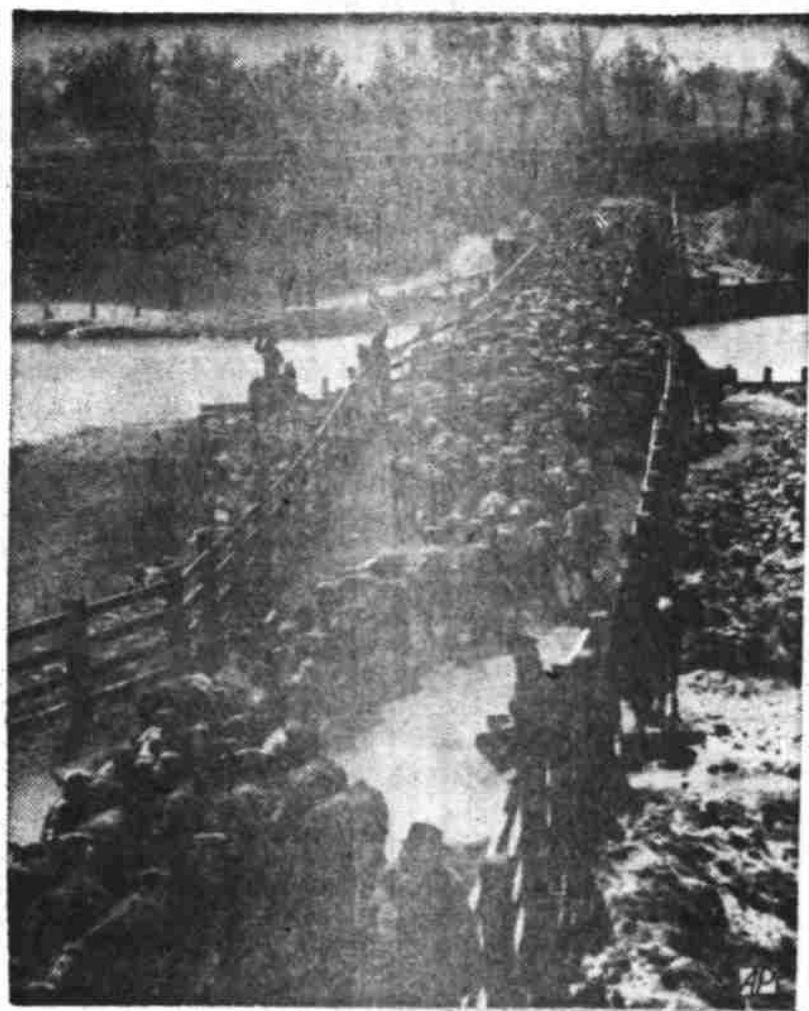
CATTLE BRIDGE OPENED —Cattle from Mexico stream across the Cordova Island bridge at El Paso, Tex., when the bridge was opened. It was constructed by cattle growers of Mexico and El Paso stockyard owners to eliminate traffic jams on the Stanton Street vehicular bridge in El Paso, where livestock have crossed previously. Both sides of the river in this scene are Mexican territory, looking south. Cordova "Island" is an arc of land jutting into the U.S. north of the Rio Grande. Ed Ardoin of the Babicora Development Co., El Paso said these cattle were from the Babicora Ranch in Chihuahua owned by William Randolph Hearst, and were destined for feeding pastures in Texas and New Mexico. (AP Photo).
