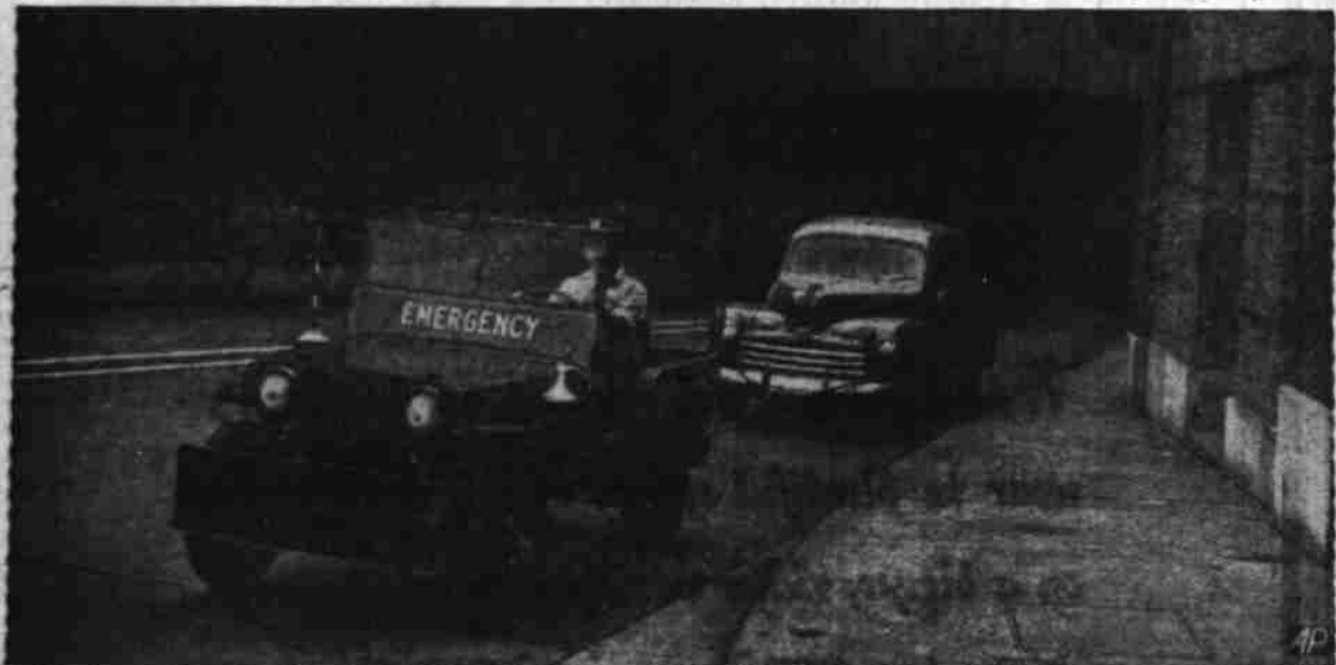
SOS SERVICE IN TUNNEL - To prevent jams in the Lincoln tunnel, handling 30,000 cars daily between New York and New Jersey, civilian jeeps tow out disabled motorcars.
