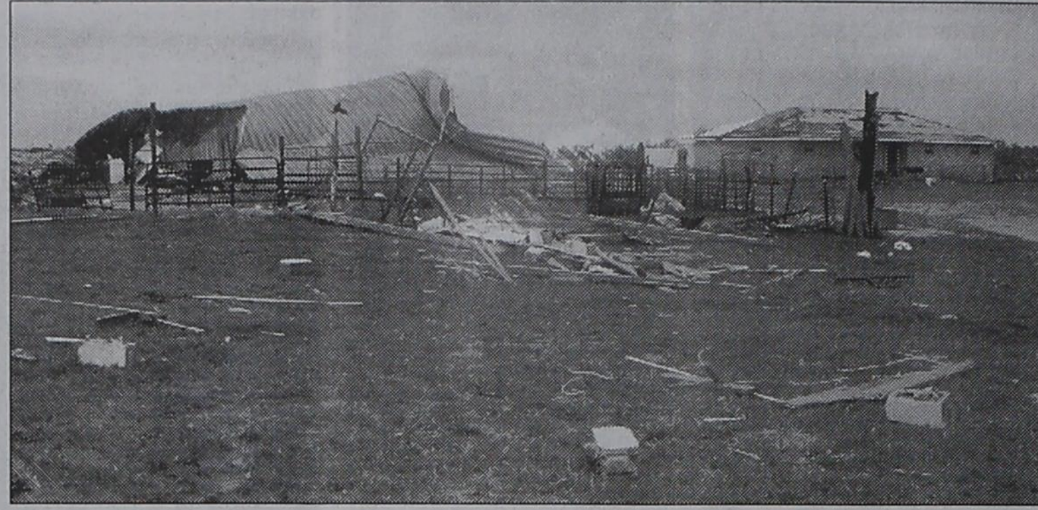
TORNADO: Wheeler county was on the weather map quite a bit Thursday evening as a storm front moved across the county. Pictured above is the home of Dean and Marla Lax; the location is two miles south of Kelton. It was reported the home is to be bulldozed down. The home of Mr. and Mrs. Matt Moore, a neighbor's house across the road north, was also unroofed. A record was set for the number of tornadoes reported in 24 hours for the Texas/Oklahoma area; 20 were reported in the Texas and Oklahoma panhandles and 26 over the entire area. The last of the clouds moved out of Wheeler county a little after midnight.
