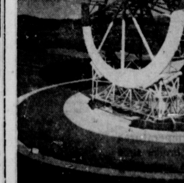
EAR INTO SPACE —This is an artist's drawing of the world's largest radio-telescope, now under construction by the U.S. Navy near Sugar Grove, W.Va. The instrument's aluminum reflector dish will have a diameter of 600 feet, twice the length of a football field. The scope will be able to pick up radio signals from space 19 times the distance probed by the 200-inch optical telescope at Mt. Palomar, Calif. Note comparative size of vehicles on roadway.
