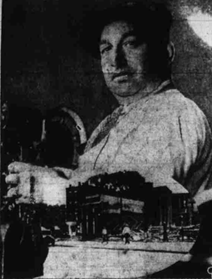
Giacomo Como, proprietor of a dilapidated cobbler's shop, inset, in a building being torn down to make way for Yale university's great medical center in New Haven, Conn., has refused to vacate until his lease expires in 1932, holding up construction.
