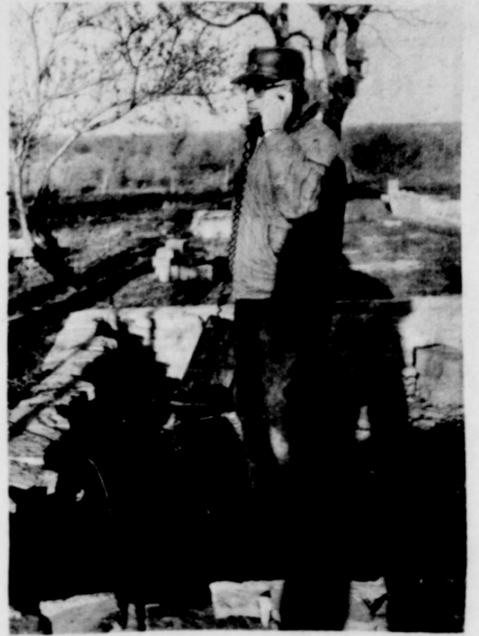
Jack Brown answers the only thing that was still in working condition following the twister which totally demolished his new home and heavily damaged the other. (Staff photo by Steve Haines).
