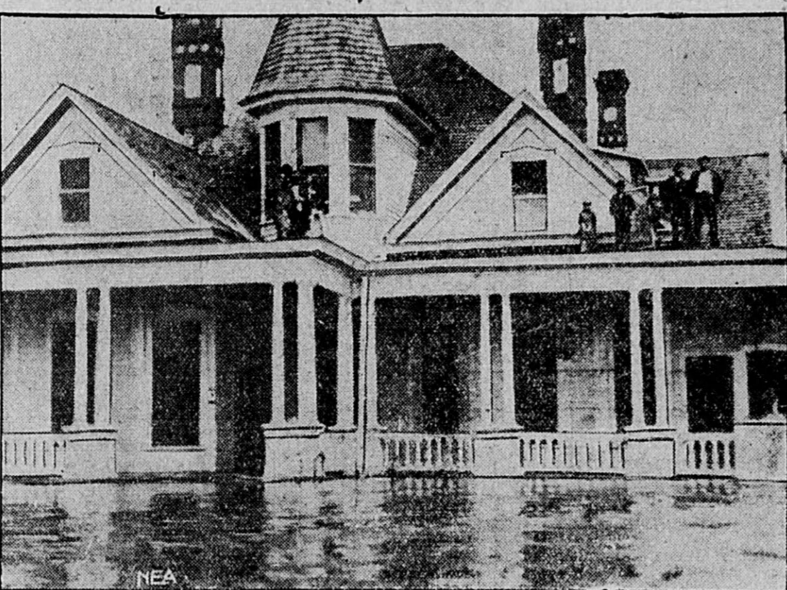
This building, the home of the probate judge of Coffee county, Alabama, at Elba, housed refugees on the upper floors for three days before relief came. This picture was taken by NEA Photographer Fred Powell; immediately after he had snapped it he brought his boat up to the veranda and began taking the refugees (shown on the porch roof) away to safety.
