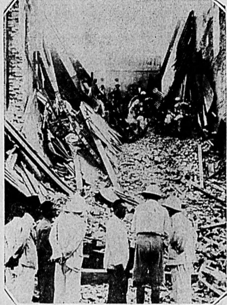
Scenes of desolation and ruin like that shown above followed disastrous earthquakes in Burma, India. This picture, taken immediately after the violent shocks, shows how an entire street was blocked by the collapse of a building in Rangoon, where scores were killed and injured. Property damage was estimated at millions of dollars. Pegu, the capital of Burma, was virtually destroyed by the quakes.
