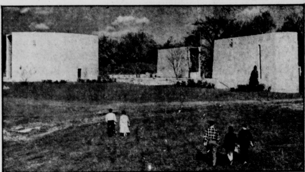
TO EACH HIS OWN —Students approach unique on-campus religious facilities of Brandeis University, Waltham, Mass. The three modernistic structures house chapels for each of the major faiths represented among student enrollment. Believed to be the only such installation in the United States, it includes, from left: Berlin Chapel; (Jewish); John Marshall Harlan Chapel (Protestant); Bethlehem Chapel (Roman Catholic).
