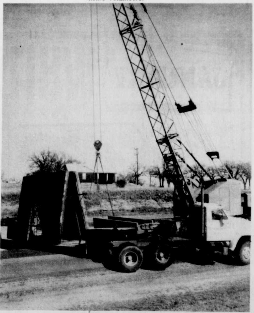
UNLOADING - - A giant crane unloads enormous pre-cast panels which are now the walls of the new lobby-chapel of the Religious Diorama at the Kendrick Amphitheater between Eastland and Cisco. The beautiful panels were brought on six trucks and installed this week.
