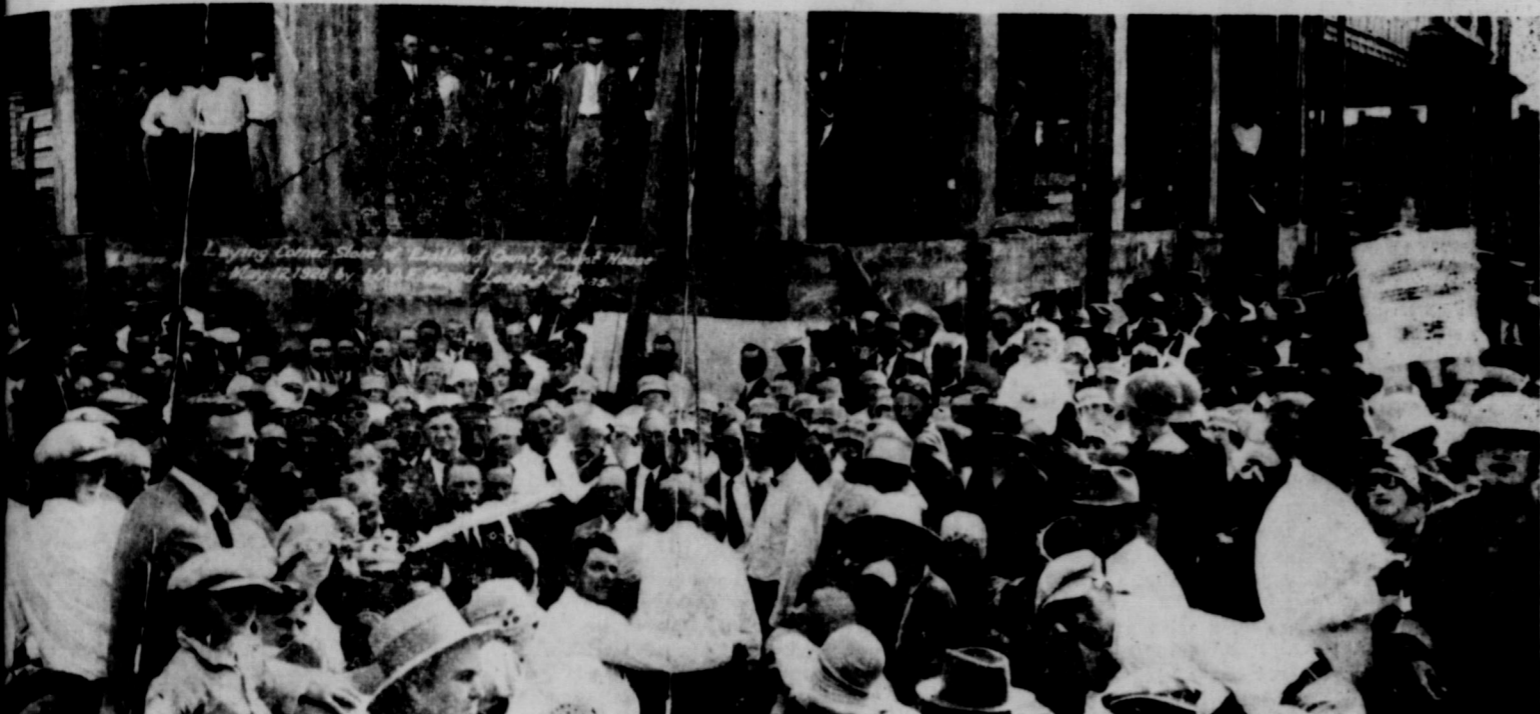
COURTHOUSE CORNERSTONE LAYING — This picture was made May 28, 1928 on the day of the cornerstone laying of the Eastland County Courthouse. The print was found recently in an old trunk and is now the property of Mrs. Everett (May) Plowman, who gave permission for its publication here. Many faces in the picture are recognized by Eastland residents. How many can you put names to?
