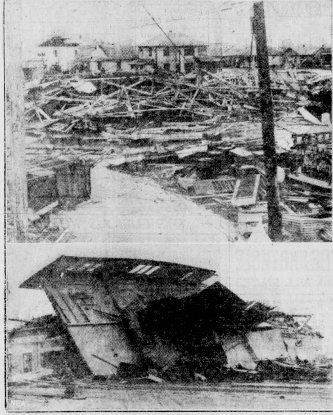
With 30 lives known lost, the hurricane which swept the Texas gulf coast Saturday night left heavy property damage in its wake. Here are two scenes showing the fury of the wind which played havoc around Freeport, Texas. Above, a section of the city showing what happened to the Ford Motor company plant, and the city's firehall. Below, a lodging house which was dumped on top of the Chevrolet Motor company.
