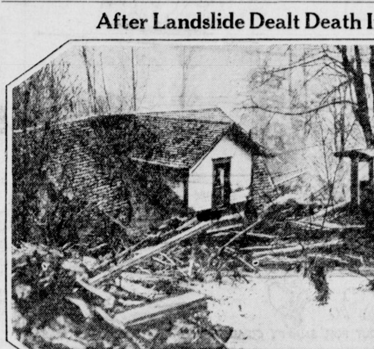
Floods of melted snow and landslides have taken a score of lives, wiped out parts of towns and caused thousands of dollars of property damage in the northwest. Here you see wreckage of the home of George Johnson, a logger, at High Point, Wash., after warm rains sent tons of boulders, logs and earth crashing down the mountainside. The water in the foreground is from a flooded creek.
