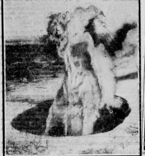
When a gas well in Refugio county, Texas, caught fire recently it immediately "cratered," forming the blazing pit pictured at the left, 160 feet long, 100 feet wide and 60 feet deep, and swallowing a 122-foot derrick and all drilling machinery. The photo of the crater was taken from the top of the derrick at the right, a neighboring duplicate of the one swallowed up in the flaming well.
