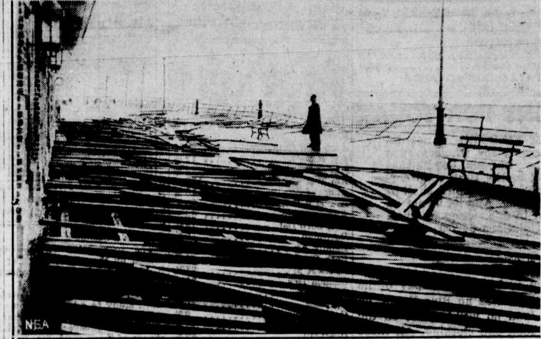
There was no strolling by honeymooners or vacationers on Atlantic City's well known boardwalk while the storm whipped at the famous New Jersey resort. Photo shows how the heavy planking was ripped up by the hurricane wave and wind.
