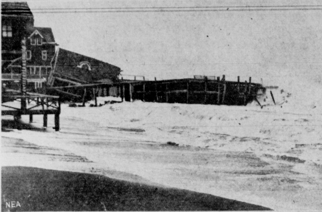
Sea Bright, New Jersey, famous shore resort, suffered heavy damage in the four-day storm that lashed the Atlantic coast. Unusually high seas pounded over the breakwater and destroyed many shoreline homes, as shown in this picture.
