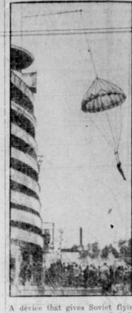
A device that gives Soviet flying students the practice needed for parachute jumping, without the risk of the actual leap from a plane, is shown here, with a pupil making his descent, in a Moscow park. The parachute is suspended, open, at 30 feet, a height where it ordinarily would not open, and then released by the device when the student is ready for the drop.
