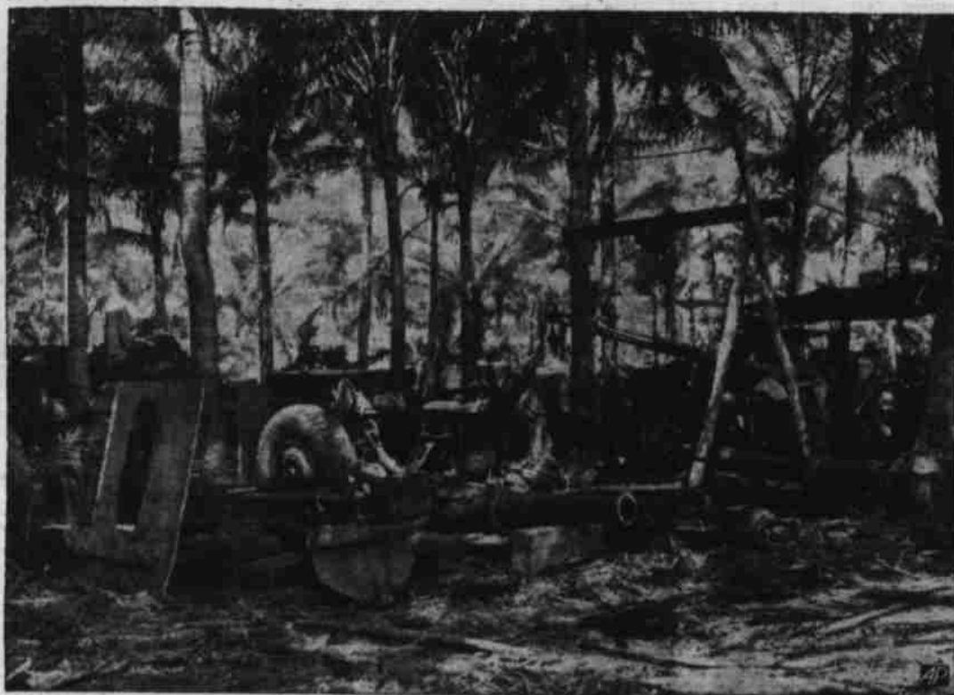
REPAIRS IN JUNGLE —As soon as the immediate area was fairly safe from retreating Japs, work started in this ordnance repair shop, erected in Wake Island jungle.
