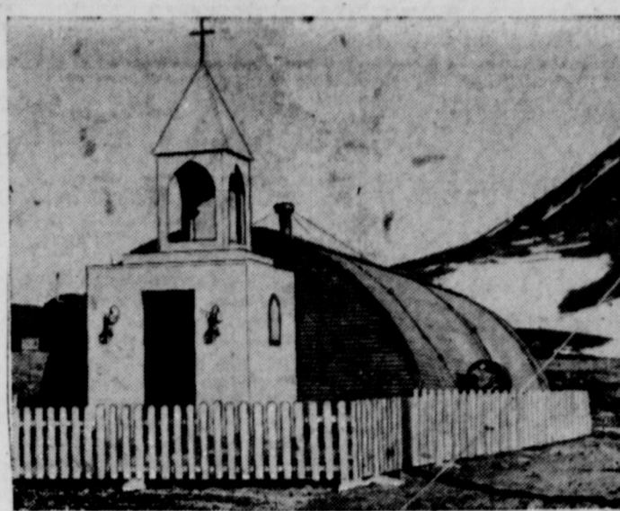
CHURCH AT THE BOTTOM OF THE WORLD —This chapel is in the deep, deep, deep South—the Antarctic. The quartz structure is at McMurdo Sound, where temperatures range near 60 degrees below zero.
