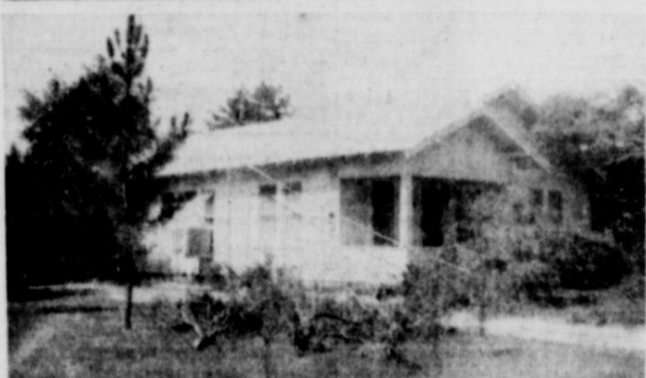
high wind at top right. The light poles on the east side of Maverick Stadium were bent over by the storm as seen in the picture at bottom left. The poles on the west side remained straight and upright. Several trees and a television antenna were destroyed at the Ray Carey's home on East Sadosa at bottom right.
