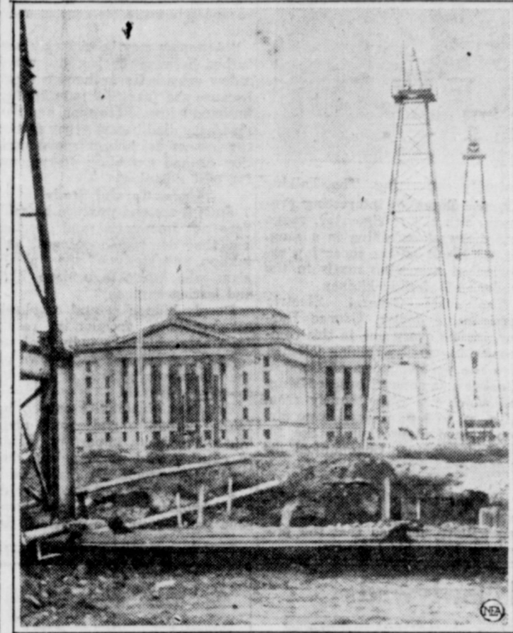
The march of the oil derricks goes on in Oklahoma City. Several of them, as pictured above, are springing up on state-owned property surrounding the capitol, latest step in the long controversy between city and state. Anxious to preserve the beauty of its capitol grounds, the city had forbidden such drilling, though private operators were permitted to drill nearby. Maintaining that the state should have the benefit of oil it owns, and that companies operating adjoining wells might drain state pools by drilling at an angle, state officials have fought for the right to sink wells on this property.
