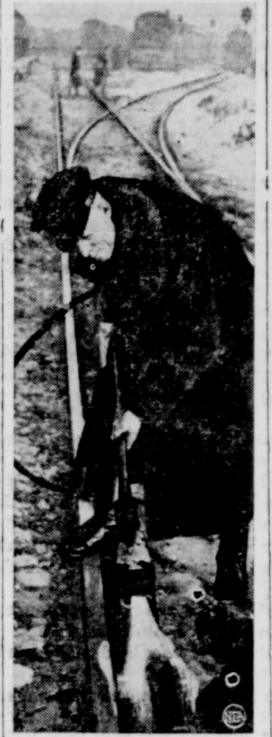
The flame-thrower wielded by the German above is not being used to destroy French railroad tracks but merely to thaw out German tracks after recent cold wave had them, causing much delay in traffic.
