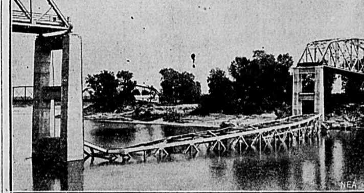
This is the scene that confronted repair crews after the new $500,000 concrete and steel highway bridge over Red river at Garland City, Ark., was wrecked by four explosions. Note how the explosives, placed under each corner of the center span, and set off simultaneously, clipped off the 305-foot section as neatly as if it had been severed by a huge pair of scissors and tossed it into 35 feet of water. Damage was estimated at $250,000. Preliminary investigation failed to establish the motive for the blast.
