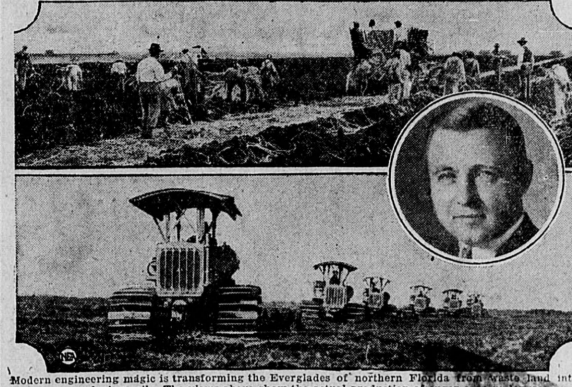
Modern engineering magic is transforming the Everglades of northern Florida from waste land into rich sugar producing soil. The views above show the actual production of sugar cane under way on a 40,000-acre tract. Drainage was effected by building a dike 31 miles long and installing gigantic pumps with a capacity of 180,000 gallons of water per minute. The pumps are reversible so the land can be irrigated in dry seasons. Soon a third sugar mill with a capacity of 3000 tons of sugar a day is to be built at Clewiston, Fla. Inset is Bror G. Dahlberg, head of the project.
