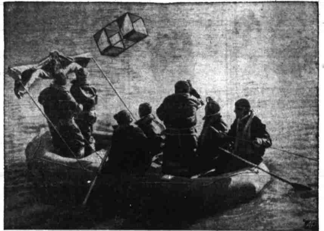
BOX KITE AIDS RAFT'S RADIO —Demonstrating equipment for downed airmen, U. S. fliers row a rubber boat and send up a box kite antenna for their radio near Bolling Field.
