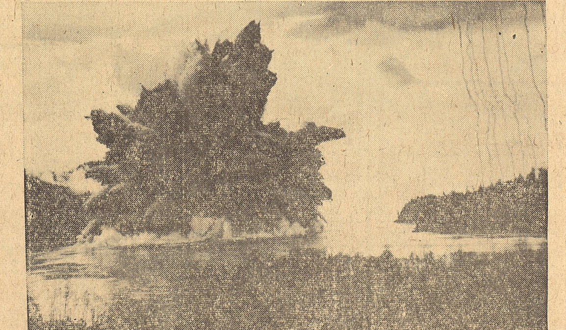
DREADED MARINE HAZARD DESTROYED—Water and shattered rock erupt from the effects of 1,375 tons of explosive, one of the largest, non-nuclear blasts in history. The Canadian Department of Public Works set off the explosion to level Ripple Rock, an underwater hazard in British Columbia's Campbell River that has claimed over 100 lives and destroyed about 120 ships in the past 100 years. The three-million-dollar project was designed to shatter about 370,000 tons of rock. Wavy lines at right are from rockets fired by scientists testing the explosion's force.
