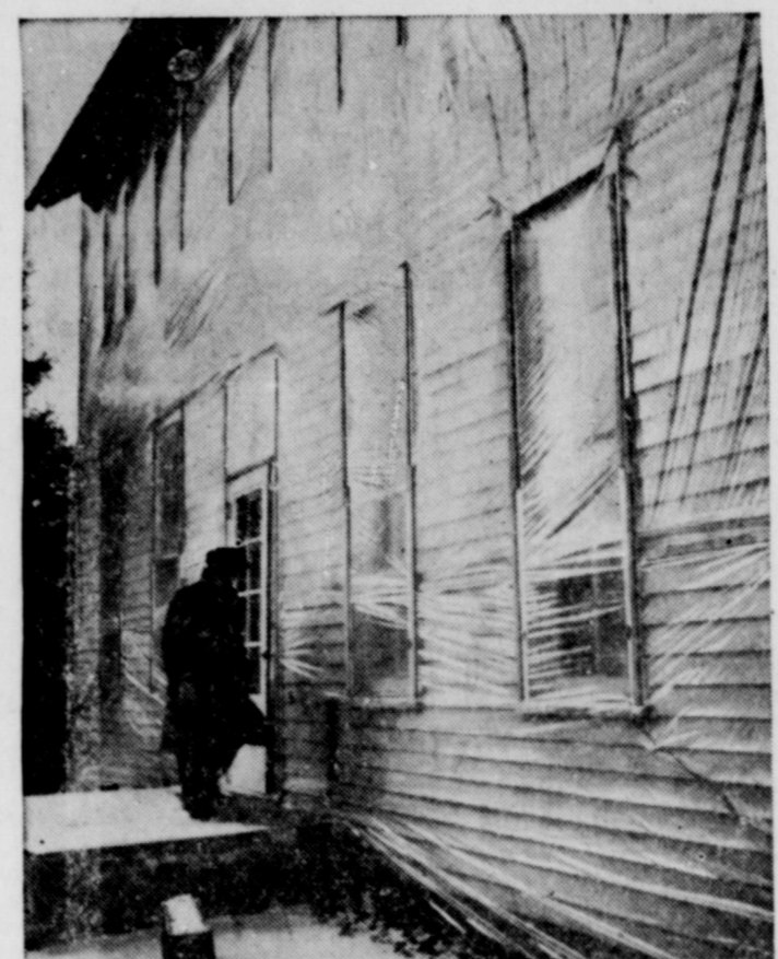
WRAPPED FOR WINTER—Wrapped in shimmering polyethylene, this old house in Lafayette, Ind., is the result of one cold winter night when the temperature fell to 10 degrees below zero. The goldfish bowl in the living room froze over, despite the fact that the oil burner was on. Purdue University Agricultural Experiment Station suggested wrapping the poorly insulated building in polyethylene film. Agricultural engineers are still testing the temperatures inside and out, but the residents of the house have been able to turn down the oil burner at night, even in coldest weather.
