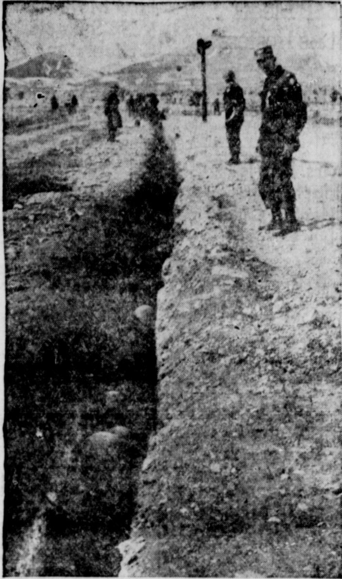
11-HOUR MINUS ONE —U.S. Army soldiers rehearse moving into trenches in preparation for D-day at the Atomic Energy Commission's Nevada Test Site. They will be in six-foot deep trenches, approximately 4,000 yards from Ground Zero at the moment of detonation, then will walk through the blast area to see the damage inflicted on equipment that stood exposed to the radiation.
