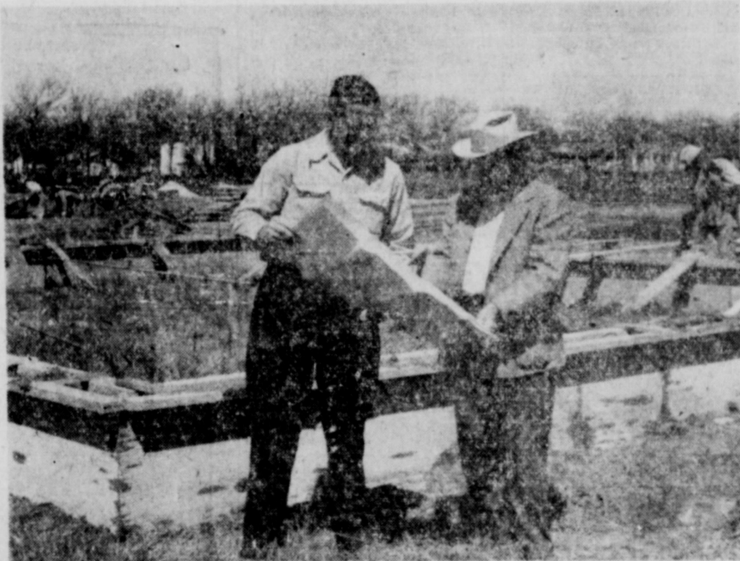
LOOKING OVER PLANS —C. C. Broyles, right, and James Dabney look over plans for a new two-bedroom home. In the background a foundation for another home in the Rivercrest Addition is going down. Broyles is contractor for the homes and Dabney is acting as local real estate dealer. Both said that as many homes would be built in the Addition as people demanded. The houses can be financed through FFA or by conventional loan. (Telegram Staff Photo)
