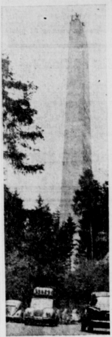
UP WE GO—Work continues on a new road between Austria and Italy, replacing a winding, dangerous highway. This column, 240 feet high, will help support a bridge.
