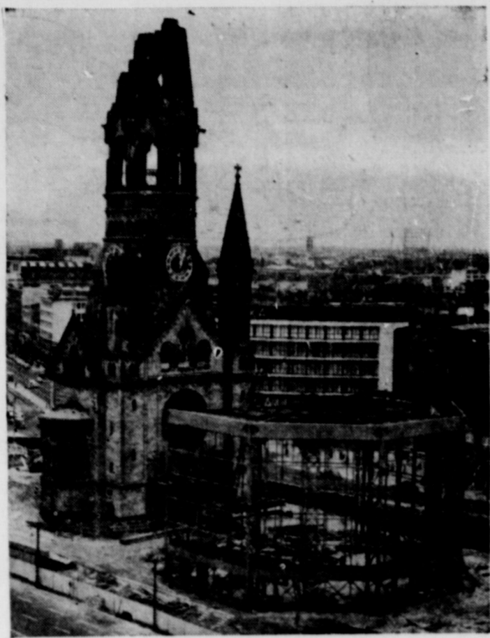
MEMORIAL FOR PEACE —West Berlin's most famous post-war landmark, the burned-out tower of the Emperor Wilhelm Memorial Church, dominates the skeleton of a new church rising in the foreground. The structure will be octagonal, with colored glass plates. The ruin will be left standing as a warning memorial to World War II.
