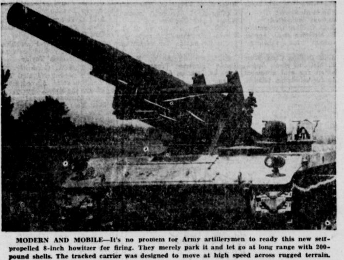
MODERN AND MOBILE—It's no problem for Army artillerymen to ready this new self-propelled 8-inch howitzer for firing. They merely park it and let go at long range with 200-pound shells. The tracked carrier was designed to move at high speed across rugged terrain.
