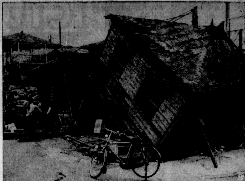
TYPHOON AFTERMATH—As soon as the roar died down from Japan's worst typhoon in many years, the residents started to repair the extensive damage. Above, people of the hard-hit town of Hakodate begin reconstruction of their wind-tossed homes, one of which is propped up by a single brace.
