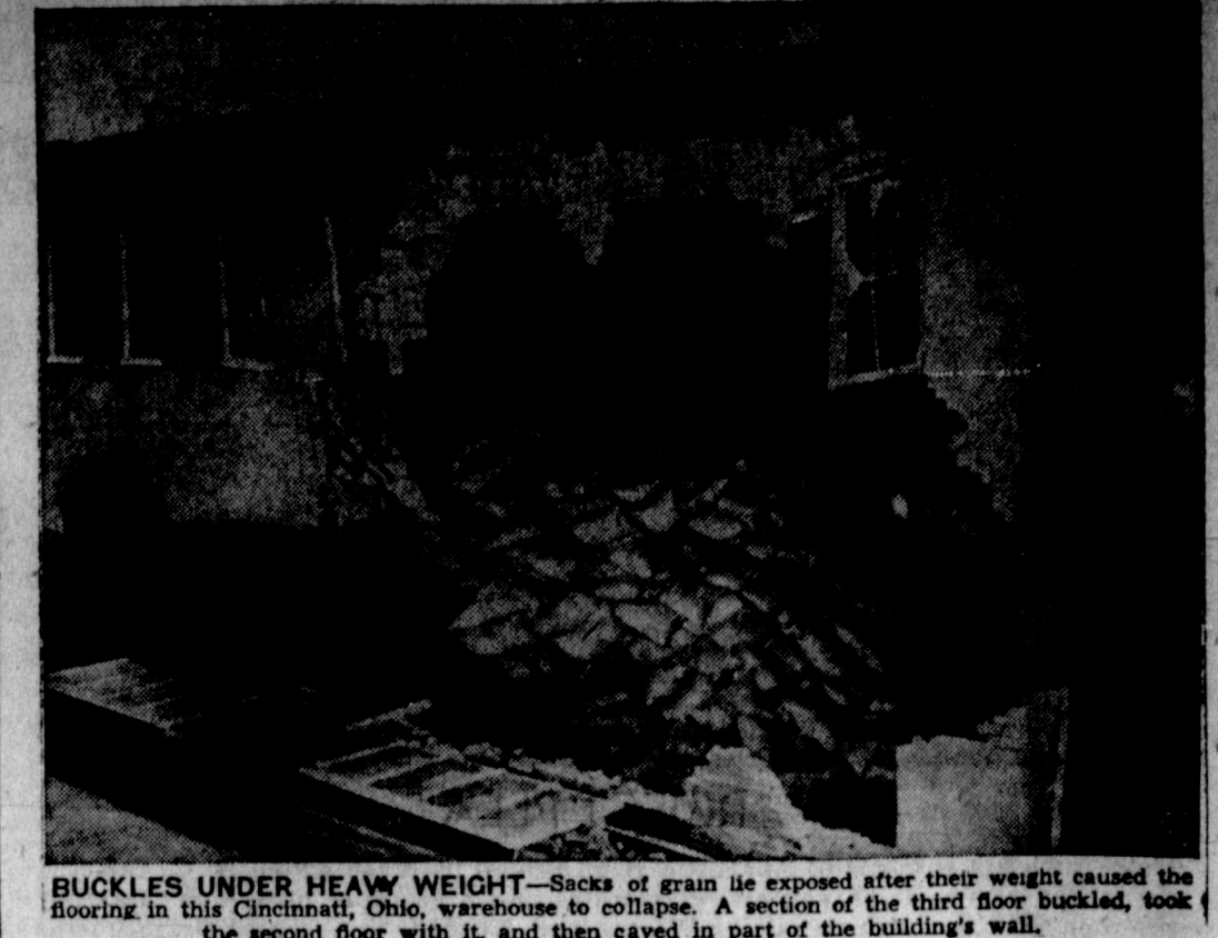
BUCKLES UNDER HEAVY WEIGHT—Sacks of grain lie exposed after their weight caused the flooring in this Cincinnati, Ohio, warehouse to collapse. A section of the third floor buckled, took the second floor with it, and then caved in part of the building's wall.
