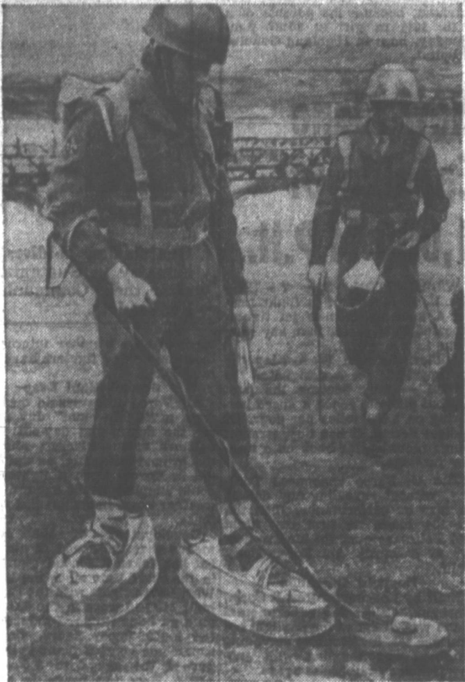
EASY DOES IT —But it pays to walk softly in a mine field, so the British Royal Engineers are experimenting with inflatable sneakers for wear in the ticklish business of sweeping for land mines. At left, sapper John Bonny inflates a sneaker before trying them out, at right. Behind Bonny is a four-footed detecting "device"—a mine-finding dog.
