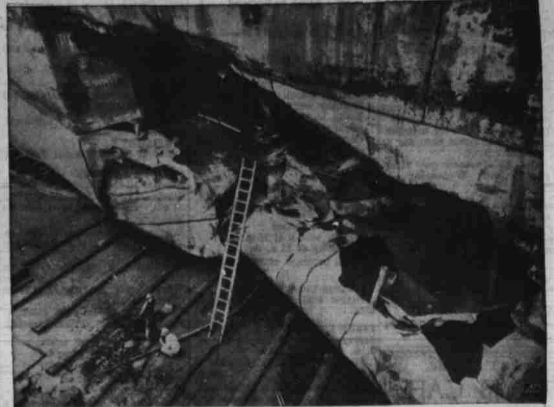
TORPEDO MAKES 60-FOOT HOLE —Shown in a U. S. dry dock, this vessel will require 1,500,000 pounds of steel to close the 60-foot torpedo hole in its bow section.
