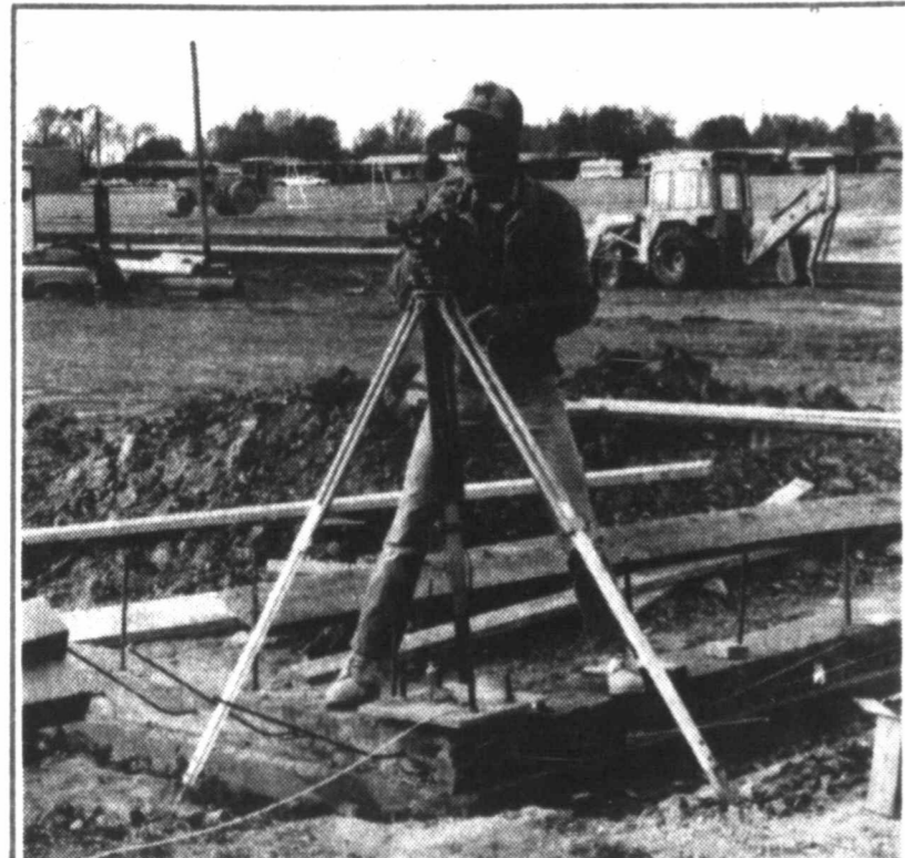
Construction workers on job
