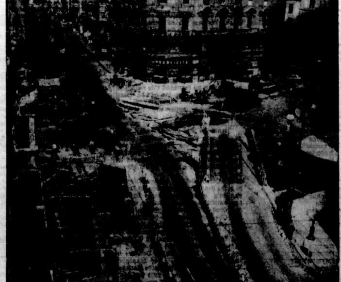
**IN A ROMAN SQUARE**—War-time Bailey bridges are being used again in Rome as the Eternal City's busiest intersection, the Largo Tritone, undergoes some modernizing. Steadily increasing traffic forced the digging up of the square and the erection of underground passageways for pedestrians. This may later be done throughout the busy city.
