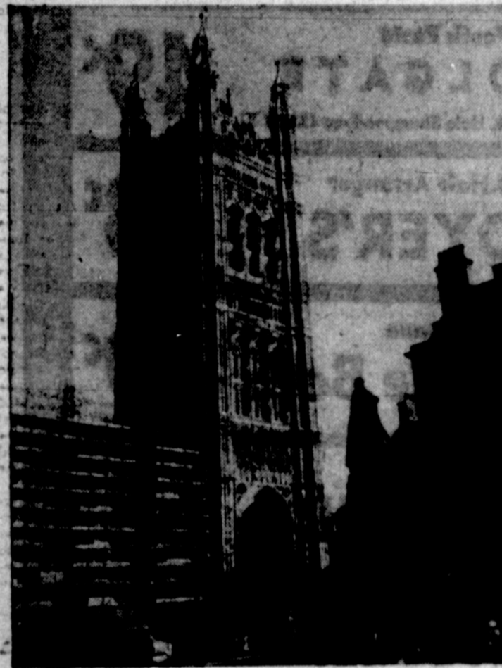
FREE AGAIN —The beautiful Victoria Tower at the Houses of Parliament in London is almost clear of the scaffolding that has obscured it since 1937. The full glory of the magnificent baroque design is now apparent once more to delight the British. In the foreground is a statue of King George V.
