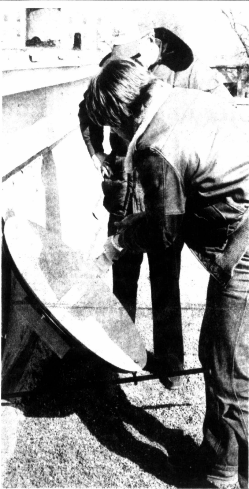
NEW TECHNOLOGY—Chris Petyan, an Associated Press technician from Vineland, N.Y., makes final adjustments to a satellite dish antenna on the roof of The Pampa News Wednesday afternoon as Morris Morgan, the
