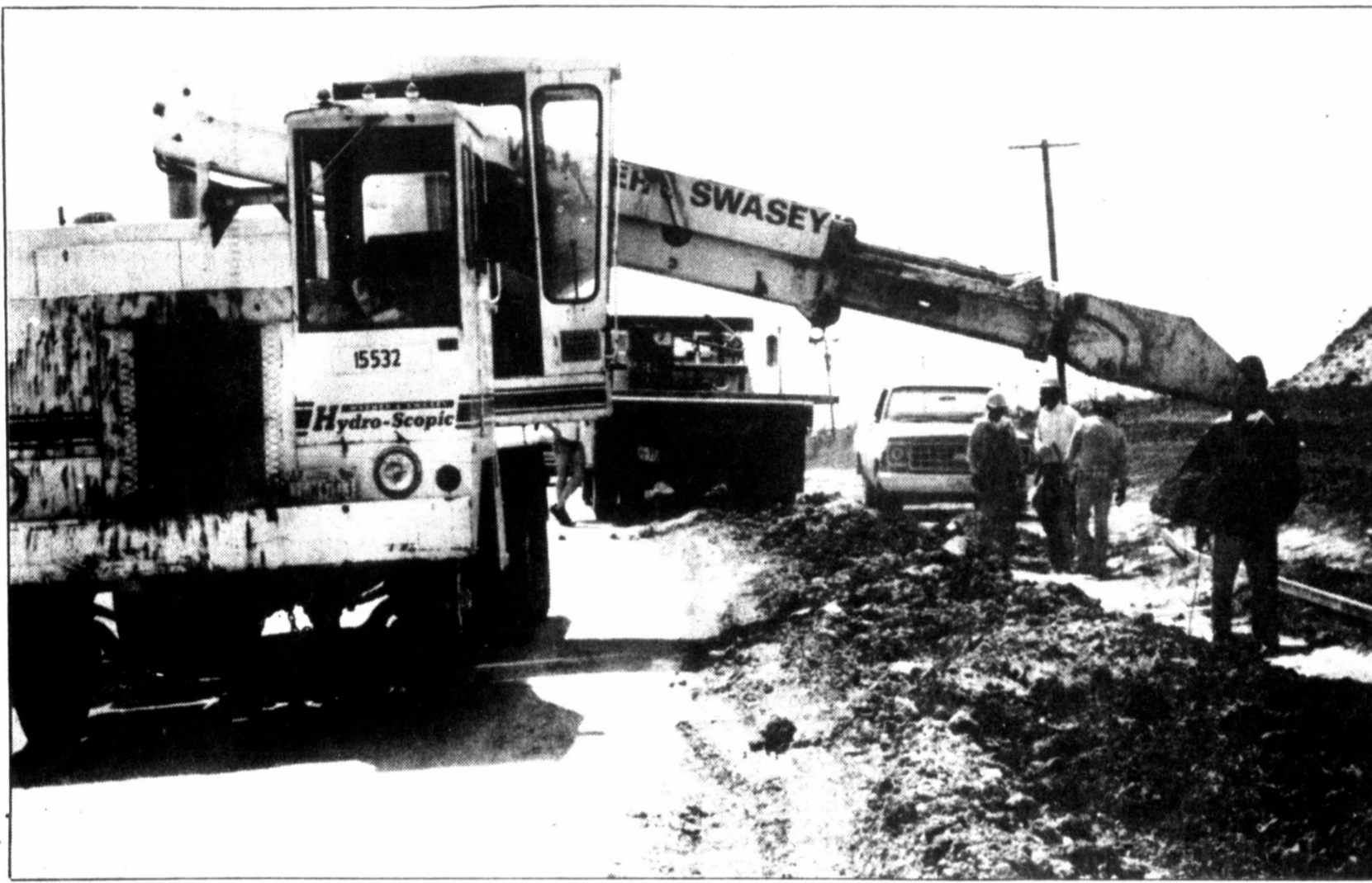
ACCESS ROAD PAVING Workers with Gilvin-Terrill, Inc., of Amarillo have been putting in cement water runoffs and grading the dirt roads circling Lake McClellan in preparation for paving projects for access roads to the lake. Double penetration seal coating will be laid on about three miles of roads connecting Hwy 70 with 140 on the north and east sides of the lake, company officials said. The paved surfaces will be 22 feet wide when completed this summer. (Staff photo by Ed Copeland)
