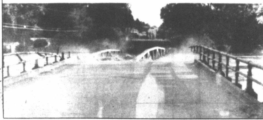
GOING, GOING, GONE —In this sequence of photographs, the U.S. Highway 6 bridge over Salt Creek, east of Ashland, Neb., was swept away by floodwaters Wednesday. In the top photo, the pavement in the foreground can be seen
