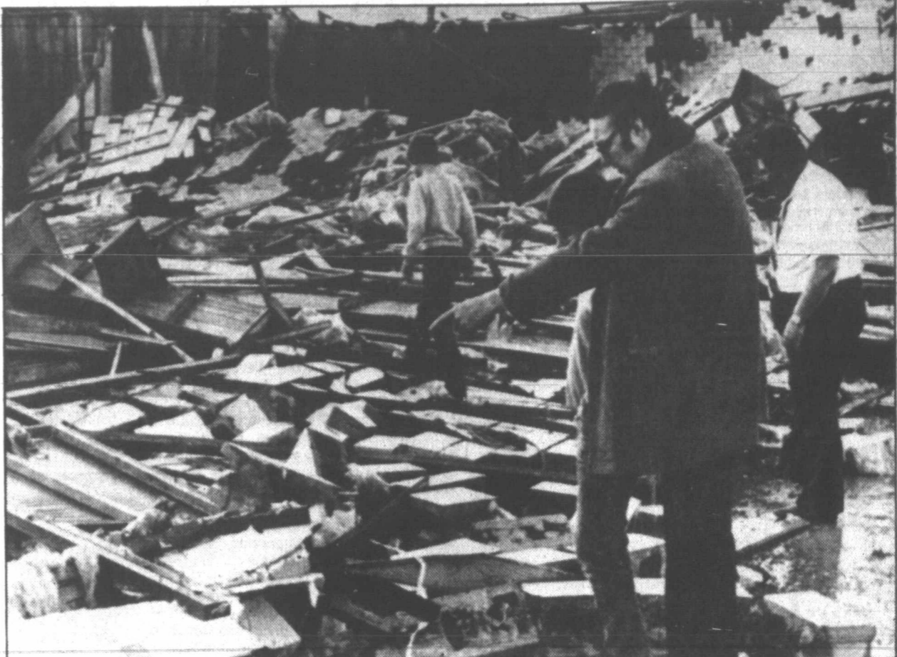
CHURCH DESTROYED—Deacon Keith Taylor, foreground, points to a crushed pew at Refuge General Baptist Church, west of Lake City, Ark. The church was leveled by a tornado Tuesday afternoon, three hours before a revival service was scheduled to start. Though no one was injured by the string of twisters that swept through the area, numerous homes and other property were damaged or destroyed. (AP Laserphoto)
