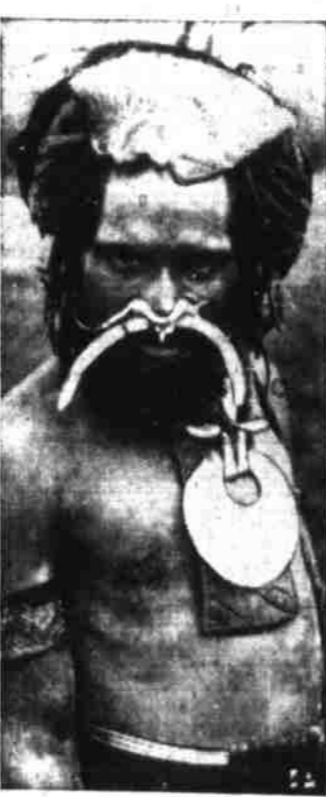
BUILDER —This ex-head hunter from the mountainous interior of New Guinea was one of numerous tribesmen used by Allied engineers to construct military highways.
