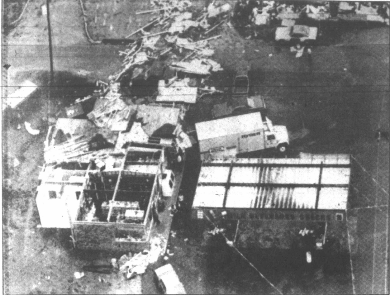
TORNADO DAMAGE —The roof of a convenience store lays scattered after a tornado blew through Montgomery, Ala., Thursday killing at least five people. Gov. George C. Wallace said he will ask President Reagan to declare the state a disaster area. (AP Laserphoto)
