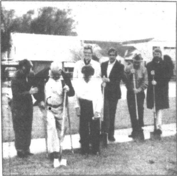
GROUND BREAKING —Members of Zion Lutheran Church, 1200 Duncan, held groundbreaking services Sunday afternoon for construction of a new annex in their church building program. From left are Robert Lemke, chairman of the building committee; J. P. and Erma Carlson, charter members of the church; Pastor Charles Paulson, and members Doug Beyer, Deck Woldst and Bill Hammer.
