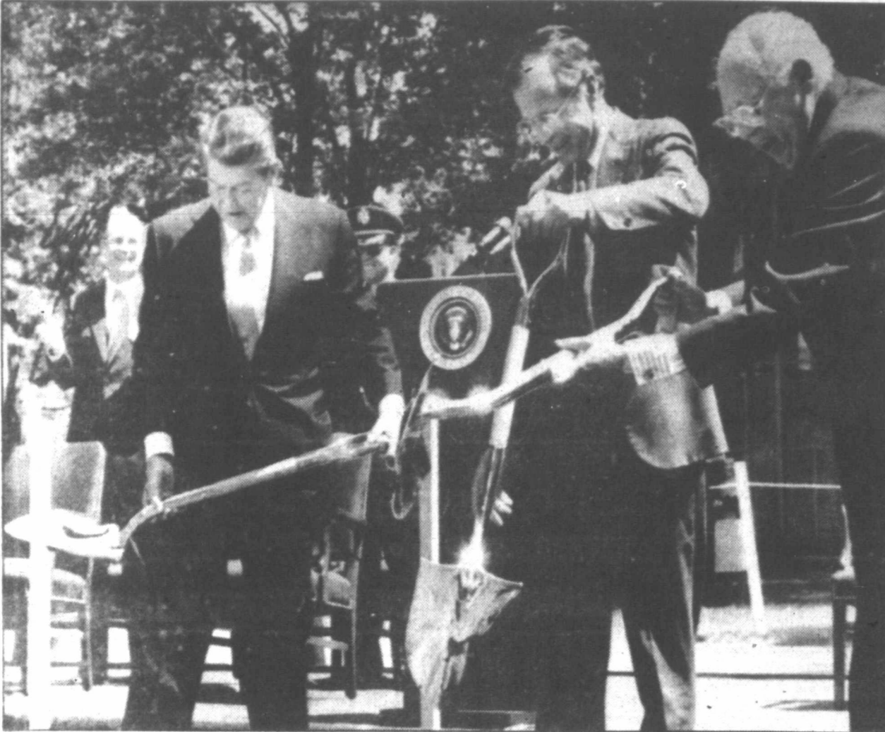
SHOVELING WITH THE CHIEF—President Reagan, Vice President George Bush and CIA Director William Casey, right, break ground for an addition to the Central Intelligence Agency headquarters in McLean, Va., outside Washington, Thursday. The 1.1 million square foot addition will double the size of the CIA headquarters.
