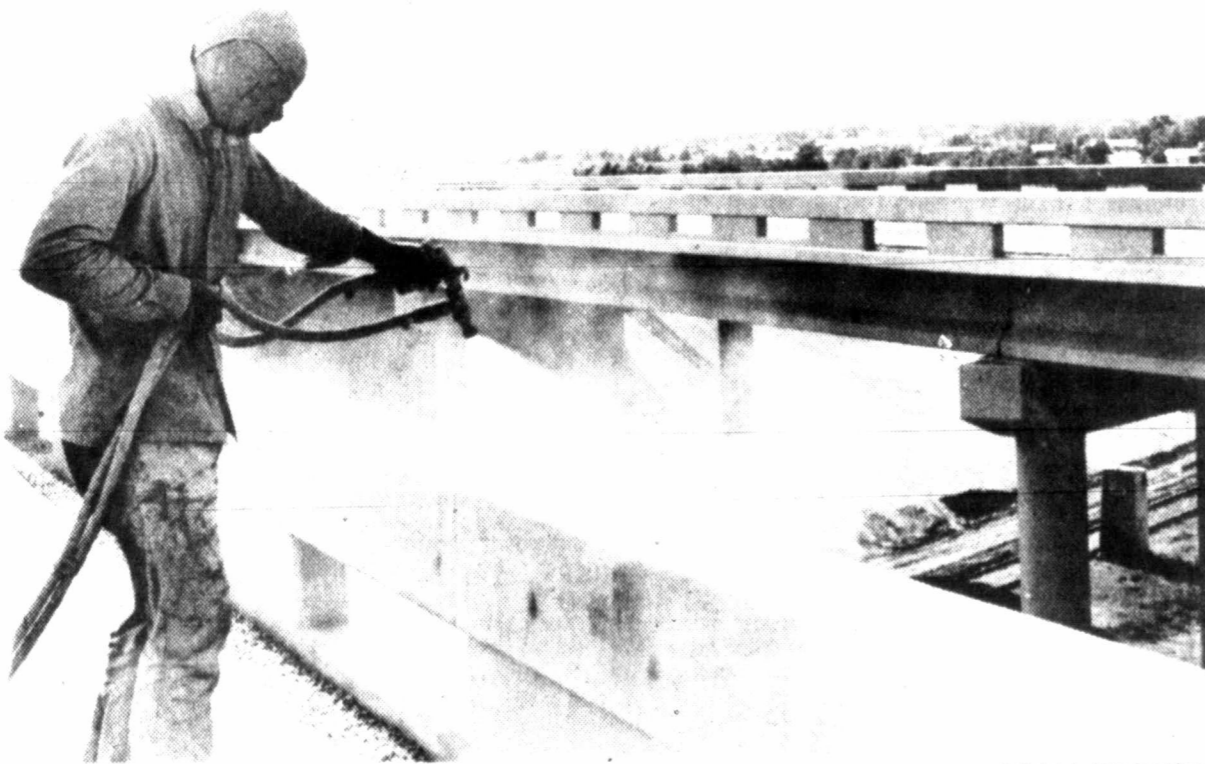
Worker paints guardrail along I-40 near McLean.
